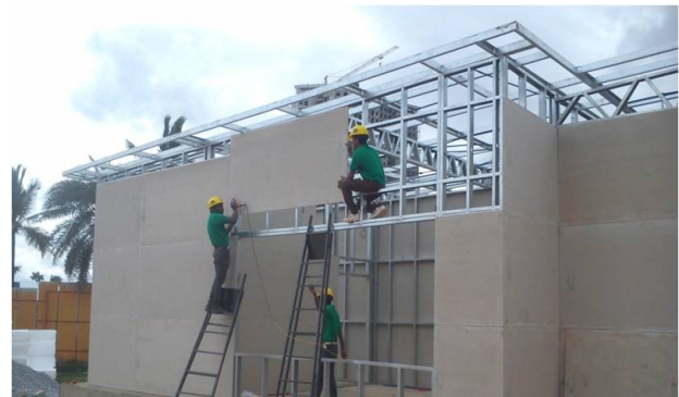
Figure 02: Fixing of outside CFBs
