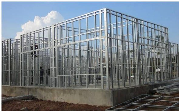
Figure 01: Erection of LGS wall frames
