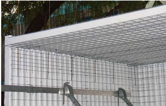
Figure 01: Reinforced EPS core panel walls and slab
