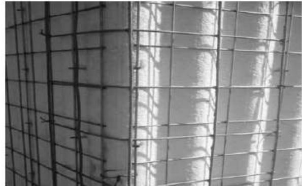
Figure 02: Corner detail in EPS Core Panel System
