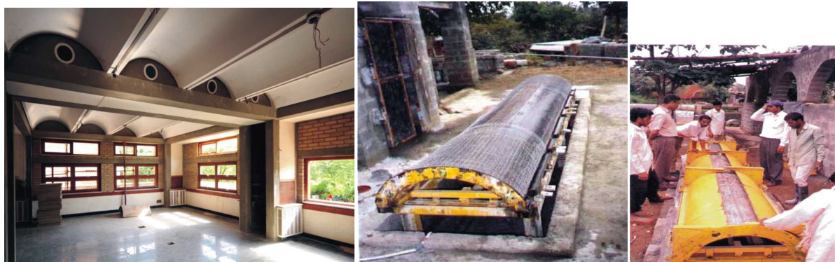
Figure 01: Construction of FC Roof channel
